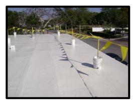
The asphaltic products, such as built-up roofing and modified bitumen make up the majority of the market but vary widely in lifetime viability – mainly because there is such a variation in the number and types of plies installed, as well as the capsheet used. APP modified bitumen will usually outlast traditional built-up roofing by at least 5 years – more if you apply additional layers.
